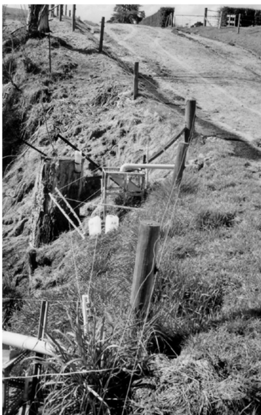
Figure 1. Picture showing one half of the road with ACH-altered slag and tipping bucket installed. Note the Mangakino stream tributary flows through a culvert located beneath and between the two tipping buckets.
