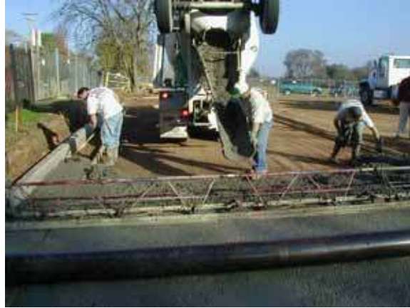
Figure 3. Vibratory screed used in placing PCPC
