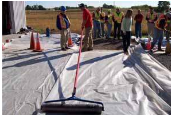
Figure 4. Transverse steel roller over the moisture barrier
