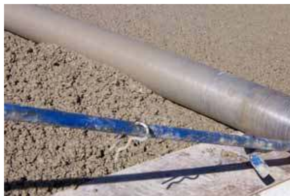
Figure 5. Compaction and finishing using a roller screed
