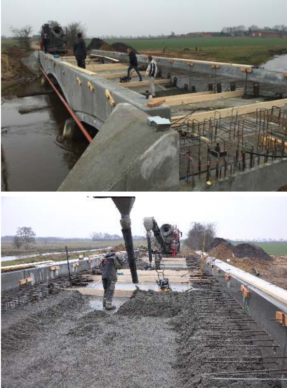
Fig. 1 PCPC cast as fill material in the very first Pearl-Chain Bridge constructed in Denmark in 2015. Upper: The longitudinal bridge section shows that the bridge consisted of a main arch between two adjacent half arches. Lower: Placement of PCPC fill. The formwork wood beams were removed as the different layers were cast.
