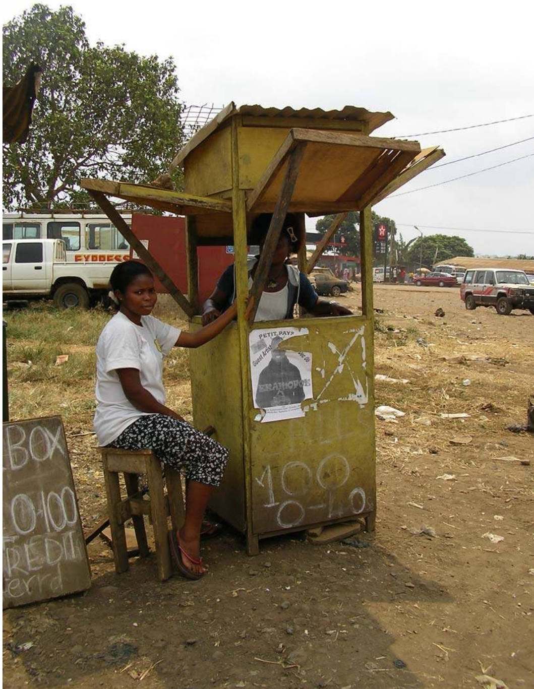
Photo 3.1 This is a typical call box. They are normally about 60x60 cm, 190 cm high and are made of timber with plywood around the lower half. They have four 'windows' that open outwards and look like wings when open. When standing inside the telephone box, only a person's top half can be seen. The roof slants and the call box can be green, brown or yellow but they are often yellow as MTN, the main mobile telephone company, has yellow as its trademark colour. These boxes are ubiquitous, omnipresent and pervasive and are rapidly changing the region's landscape/socio-scape.
