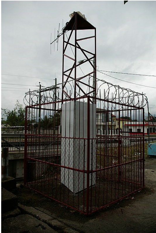
Figure 12: 5 Meter Antenna Tower for Computation Nodes
