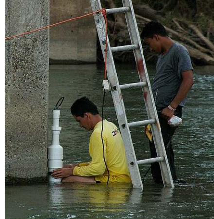
Figure 13: Installation of Water Level Prototype by FSAR Employees
