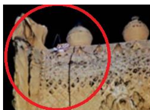
FIGURE 2. Brihadishvara Temple – Lightning strike chipped-off mortar in precincts adjacent to main tower (Sri Vimana) in 2011
