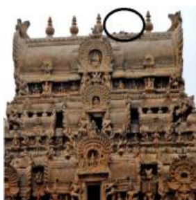
FIGURE 1. Brihadishvara Temple – Lightning Strike shattered the spire atop Rajarajan Tower (Gopuram) in 2010
