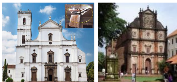
FIGURE 6. Damaged roof and gables due to lightning strikes in Se Cathedral and Basilica of Bom Churches at Goa during 2015 and 2016 respectively
