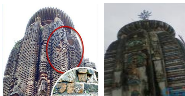
FIGURE 5. Lightning Strikes in (a) Jameswar and (b) Nilamdhab Temples respectively
