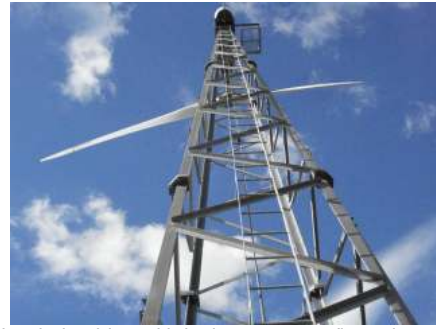
Fig. 4. Gaia wind turbine with lattice tower configuration
