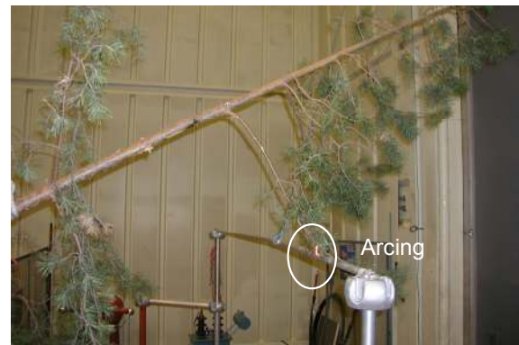
Figure 2. Arc-associated tree bending over the conductor.
