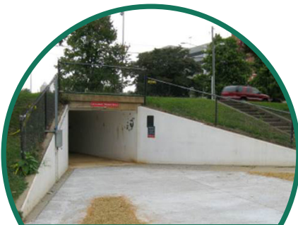
Charlottetown Dr Ped/Bike Tunnel
