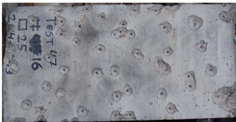
Figure 3: Damage on the top surface of a 200 mm slab. This test was as a source for the impact locations in test 1 of the FEA simulations. The image was provided by and is the property of DSTA.
