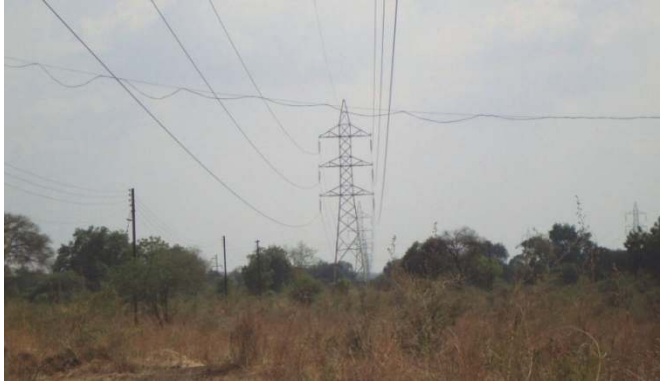
Figure 2. Site Selected for Measurement of Electromagnetic Field Emanating from Double Circuit 132 kV Transmission Line
