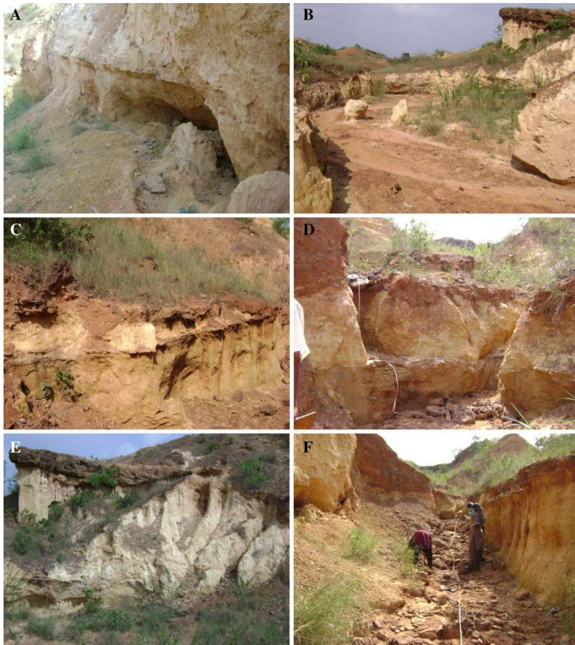
Fig. 8 Gully erosion processes in the Garbheta block. a Sidewall erosion, b gully widening, c active gully erosion during heavy rain events, d gully formed by retrogressive erosion with narrow and
