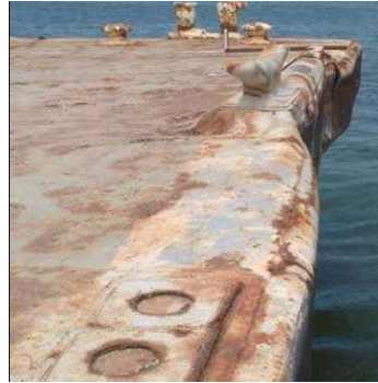
Figure 2.5 Barge bow deformation [53]
