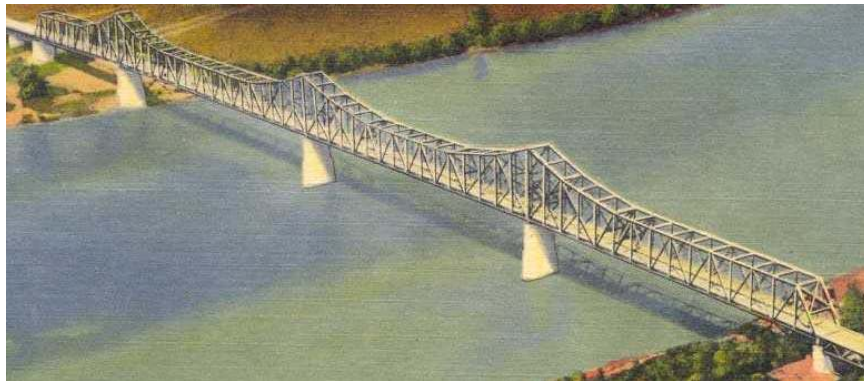
Figure 10.6 Side view of the US41 Bridge over the Ohio River
