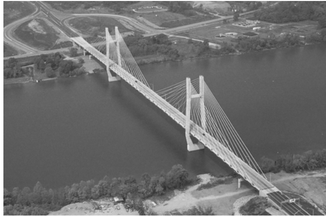
Figure 10.11 Aerial view of the Maysville Cable-Stayed Bridge
