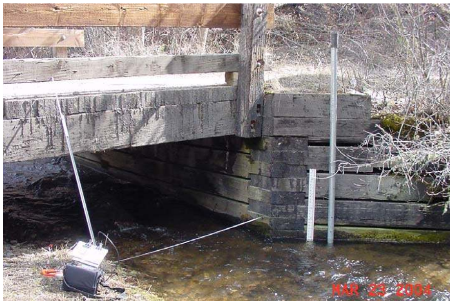
Figure 22 – DNRC AquaRod stream gage on Eightmile Creek at the confluence with Sluice Creek (Roberts, 2006).
