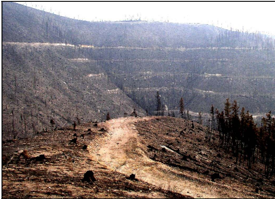
Figure 10 – Post-fire erosion hazards associated with an extensive forest road network, steep slopes, and high severity fire (Lolo Burned Area Emergency Recovery Team, 2003).
