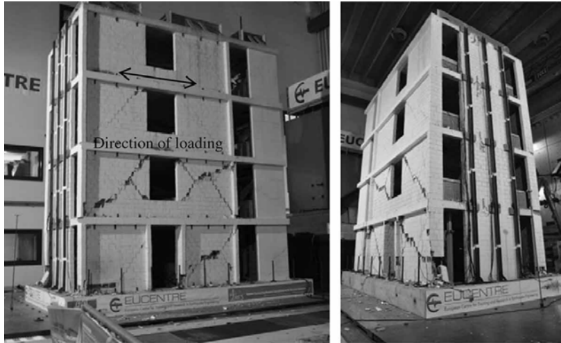
FIGURE 3 Crack pattern in a four-storey mixed RC-URM wall structure, from Beyer et al. [2014].
