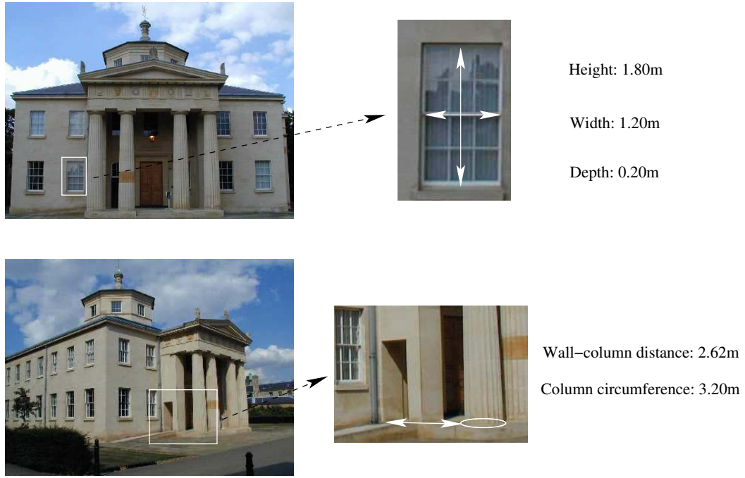
Figure 14: Some measurements made of the Downing Library scene. The other windows in the scene are the same size as the one shown (to an accuracy of \pm 1\text{cm} ).
