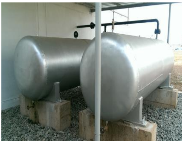
Figure 6. Settling chamber.
