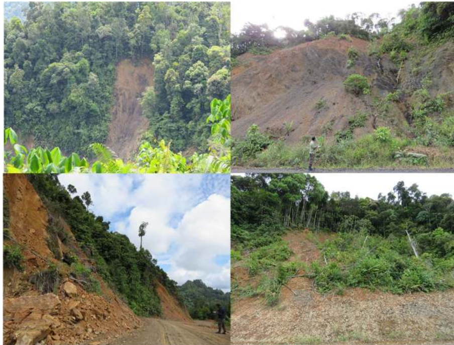
Fig. 1 Slope failures observed in the study area
