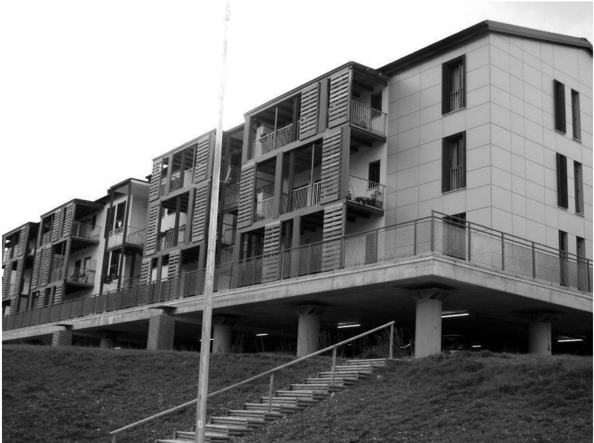
Figure 2. CASE transitional housing at Bazzano outside L'Aquila city (photo by author). The base isolation columns support the building and protect it from earthquake shaking.
