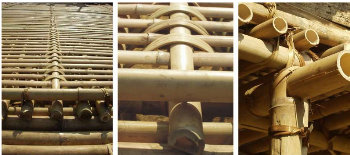
Figure 5 Work of art or innovative building technology? Photograph showing the method of clipping without nails and thongs to join loose construction members in the char (open raised terrace). Photo: authors.
