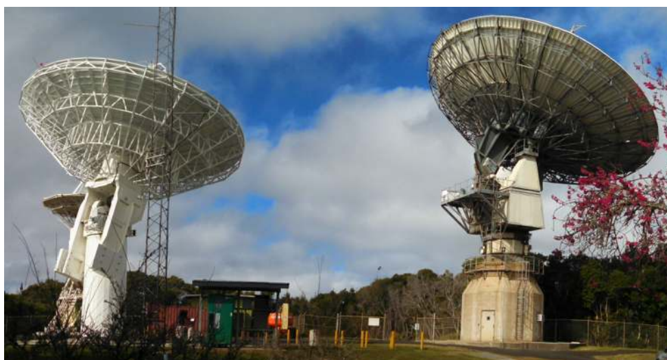
Fig. 6 New 12-m VGOS antenna at NASA's Kōke'e Park Geophysical Observatory (KPGO) on Kauai, Hawaii is shown (left) alongside the legacy 20-m VLBI antenna (right)
