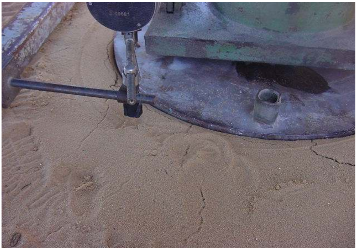
Figure C.4: A close up picture of the failure occurred in the sandy soil on site
