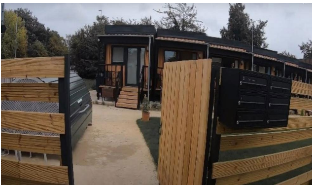
Fig. 2 Exterior view of the modular homes showing frontage, letterboxes, communal garden and bicycle storage
