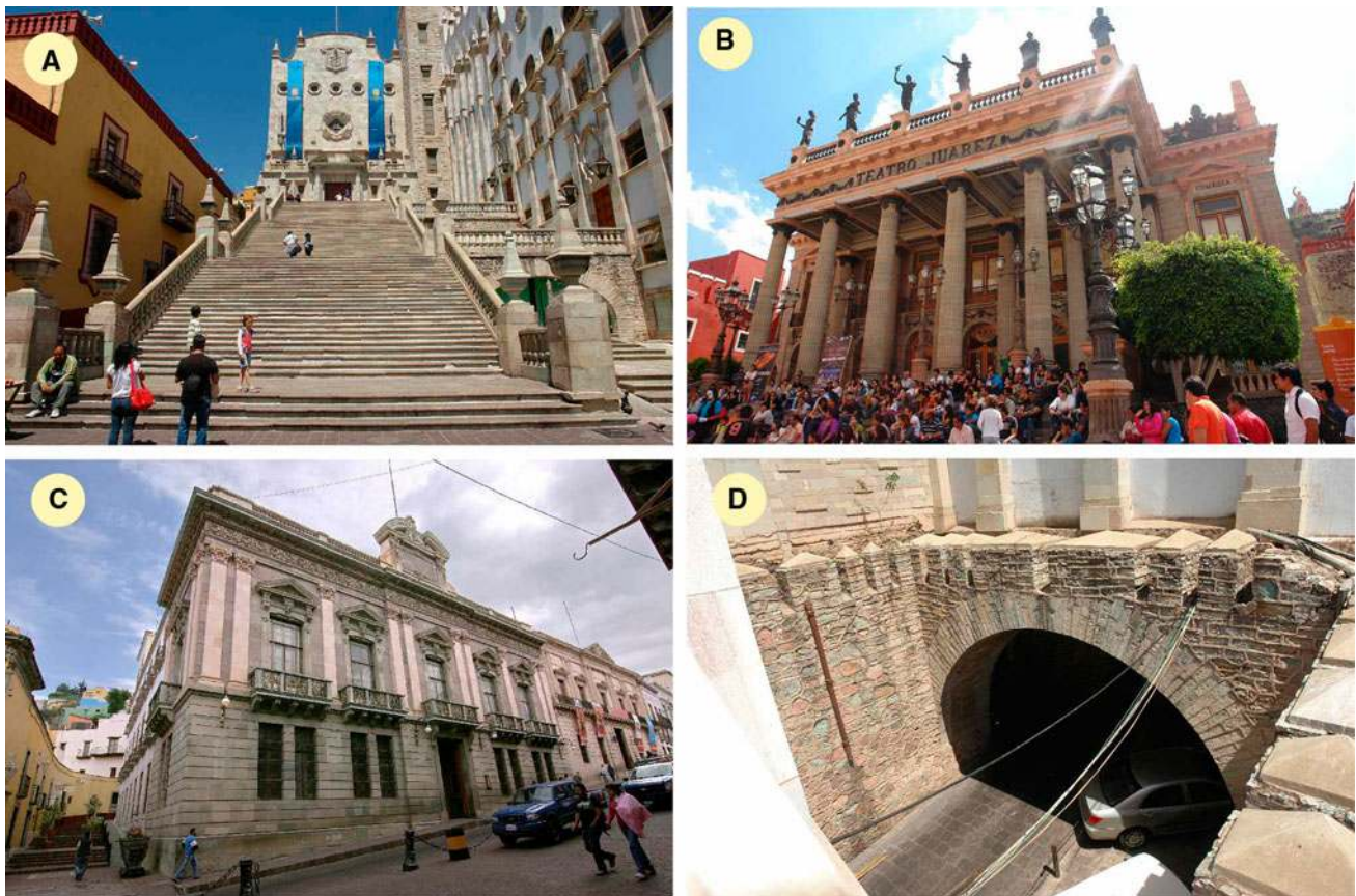
Fig. 1 Historic buildings erected with the Loseros Tuff in the city of Guanajuato. a Staircase and facade of the central building of the University of Guanajuato. b Juarez Theater in the centre of the city, the columns and the facade were built entirely with the studied tuff. c Legislative Palace whose facade is built with cuts parallel to the lamination ( X -axis) of the Loseros Tuff. d Entrance to one of the underground tunnels that cross the city
