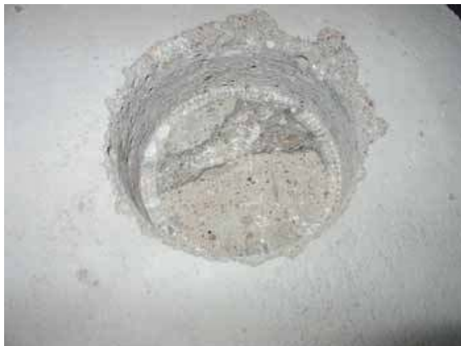
Figure 19. The remaining hole from \text{Ø } 90 \text{ mm} core drill, after extracting samples to moisture distribution determination before flooring. Drilling was performed from the top in a homogenous slab from Batch 1. Note the clear breaking zone separating the mortar screed from the concrete material.
