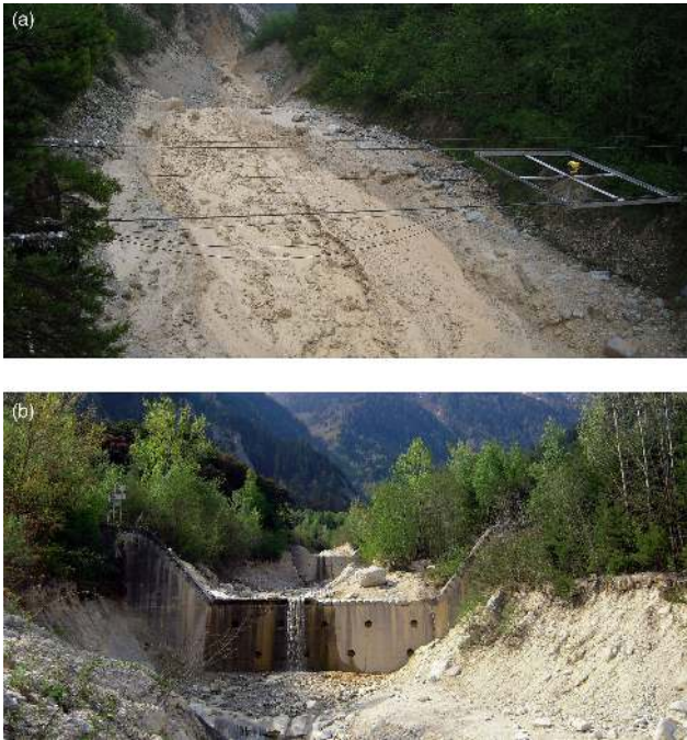
Figure 2. Debris-flow EWS Illgraben (Canton VS, Switzerland): (a) the debris-flow detection system in the upper part of the catchment (b) the lower part of the catchment with warning system.
