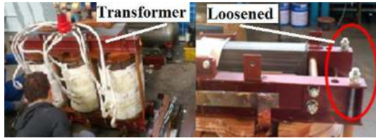
FIGURE 20. Transformer disassembly inspection experiment
