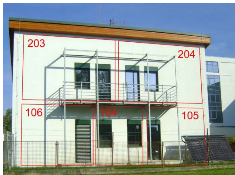
Fig. 1 Smart home—wooden house, training center of the Moravian-Silesian wood cluster (MSWC)
