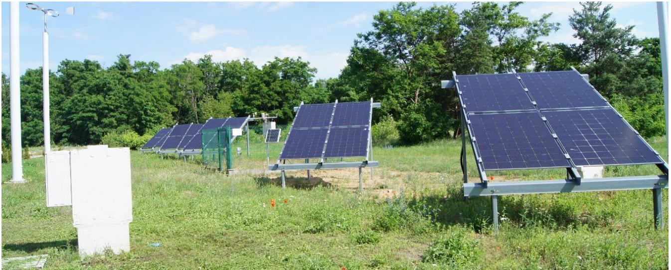
Figure 7. Setting up 5 \times 4 panels on the ground in Bydgoszcz.
