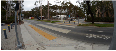
Figure 10: Intersection used to conduct the highway coverage evaluation, consisting of a two-lane driveway crossing a four-lane divided road.
