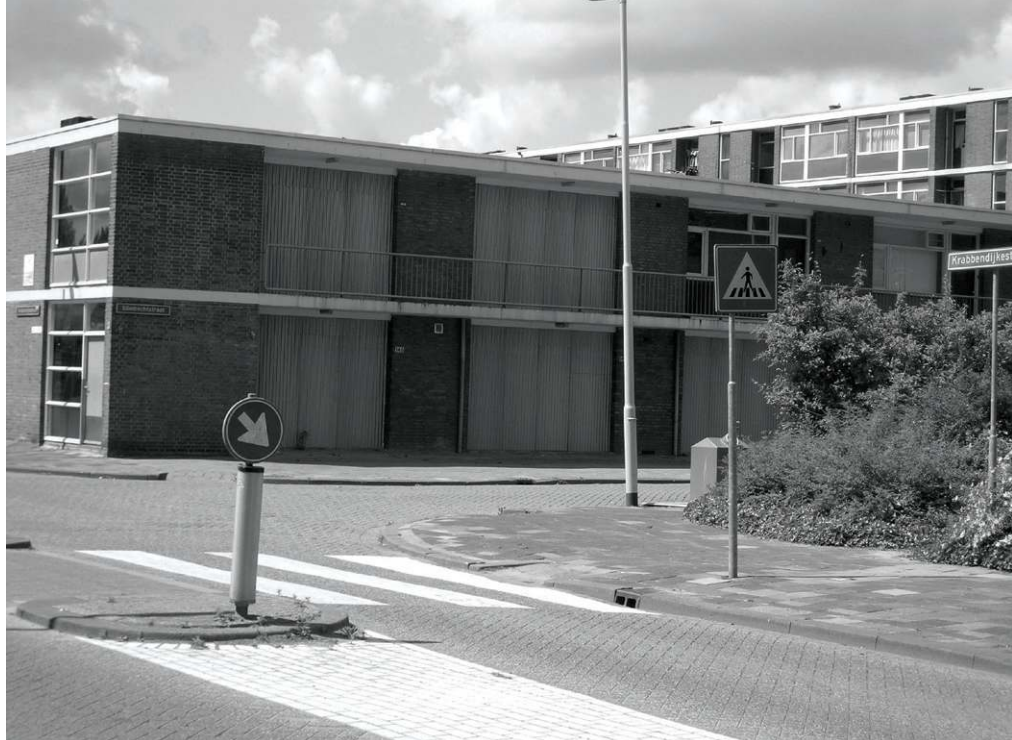
A 1960s flat in the garden city of Pendrecht, ready to be demolished in 2009, photo MvdB
