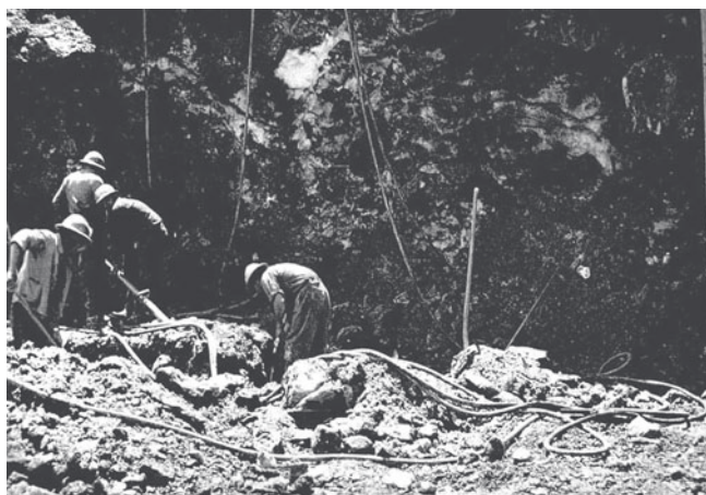
Fig. 1. Excavation of material for the construction of the Grande Dixence dam in ice-rich permafrost of a rock glacier at the locality Prafleuri, Valais Alps, Switzerland. (Photo: W. Fisch 1956; cf. Fisch and others, 1978.)
