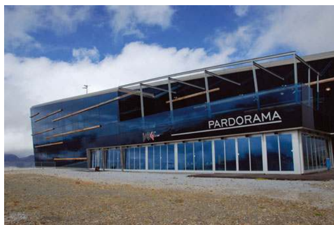
Fig. 11. Mountain restaurant 'Pardorama' in Ischgl, Austrian Alps, located at 2600 m a.s.l. in permafrost terrain. The building weighs 1400 tons. It is underlain by a three-point foundation which can be raised using hydraulic pumps; steel plates can be inserted below to compensate for settlement of the underlying substrate (currently \sim 4 \text{ cm a}^{-1} ). (Photo: M. Phillips 2010.)
