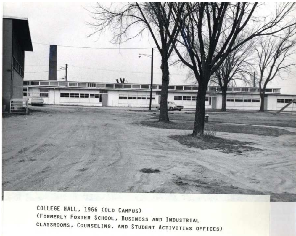
Figure 4.28. WCC campus at Willow Run Village.
