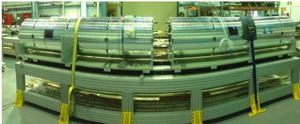
Fig. 6.21. “Panoramic” view of magnet integration table, shown with two half-length shell-yoke assemblies prior to joining.
