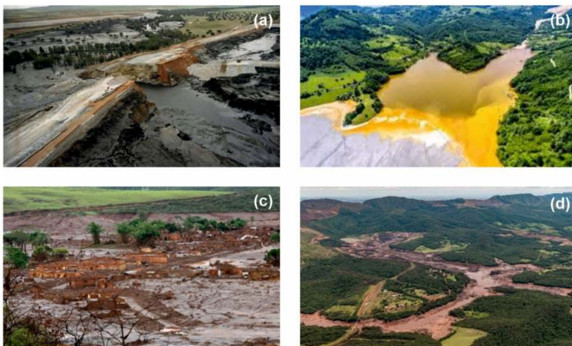
Figure 3. Images of several environmental disasters produced by collapse of tailing dams: (a) collapse of tailings dam in Aznalcollar, Spain, 1998 [22]; (b) Baia Mare disaster, Romania, 2000 [23]; (c) Mariana dam disaster, Brazil, 2015 [24]; (d) Brumadinho dam disaster, Brazil, 2019 [25].
