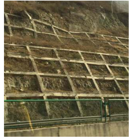
Figure 7: Concrete grids as a slope stabilization intervention
