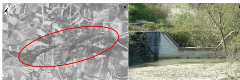
Fig. 6 Location of the remedial work visible on the historical aerial reconstruction (a); details of the concrete weirs built along the tributary of the Verrino Creek (b)
