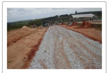
Figure 9: WBM road construction in landfill site.
