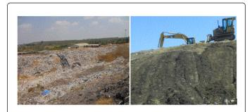
Figure 6: Typical construction procedures of soil cover.
