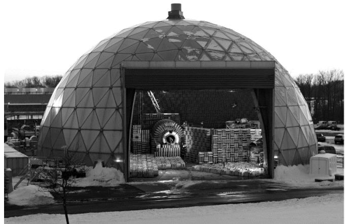
Figure 12.—Aero-Acoustic Propulsion Laboratory (AAPL).
