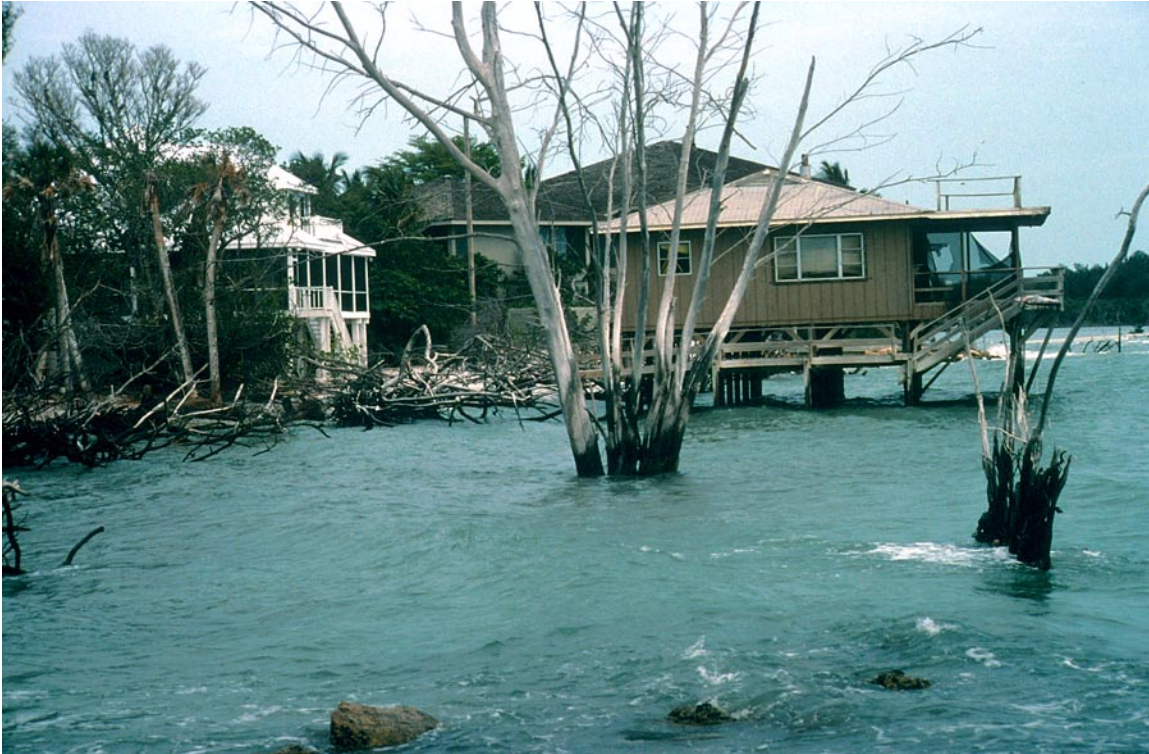
Figure 14. Erosion of the Gulf shore eventually destroyed this beach house at Captiva Island, Florida.
