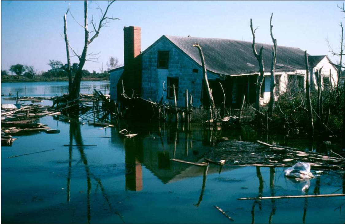
Figure 11. A coastal subdivision of nearly 200 homes near Houston, Texas was submerged as a result of subsidence induced by ground-water production.
