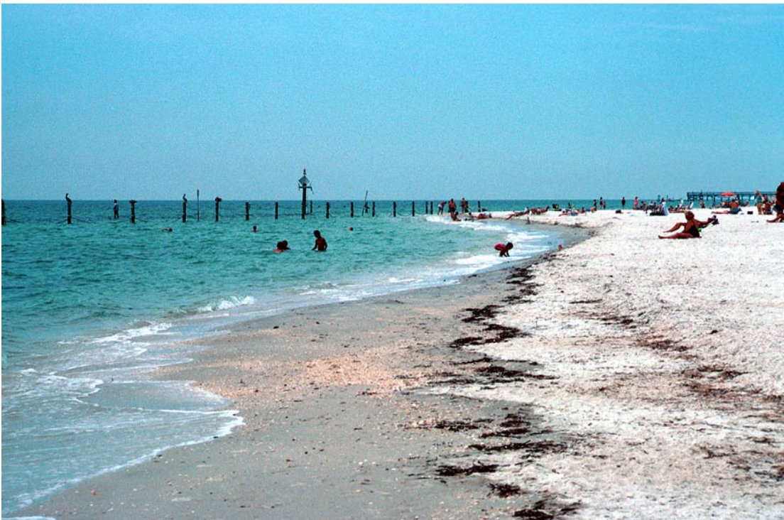
Figure 22. The breakwater at Redington Shores, Florida has protected the beach fill but has aggravated erosion of adjacent sand beaches.
