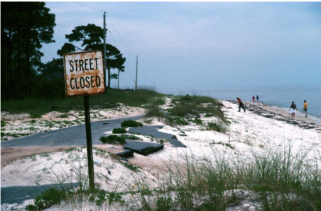
Figure 15. Even where wave energy is normally low, episodic erosion during storms is capable of destroying roads and eliminating the beach. This example of erosion along the low energy coast is from Lighthouse Point, Florida.
