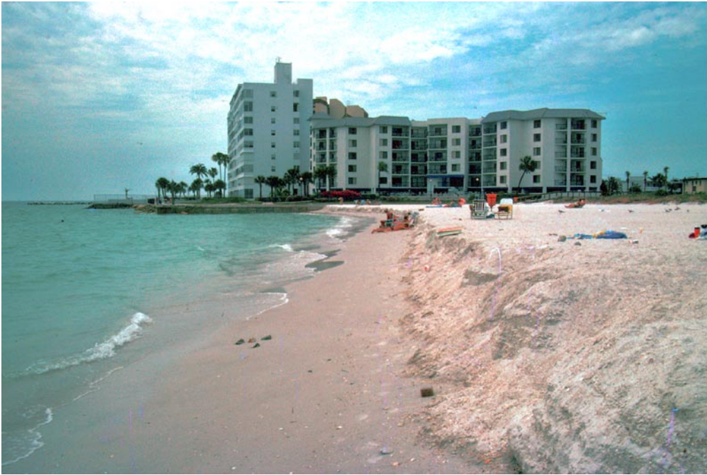
Figure 17. Many nourished beaches along the west Florida coast, such as this one on Sand Key, have steep erosional escarpments early in the history of the project.
