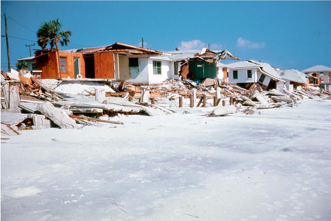
Figure 13. Property damage near Panama City, Florida caused by Hurricane Eloise in 1975. From Morton (1976).
