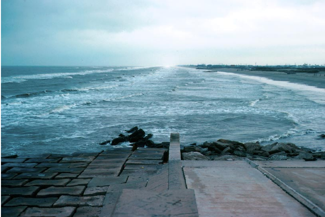
Figure 25. West end of the seawall at Galveston, Texas. The concrete ramp (right foreground) was the road leading to the beach in the mid 1960s. Since then the beach has eroded more than 150 m.
