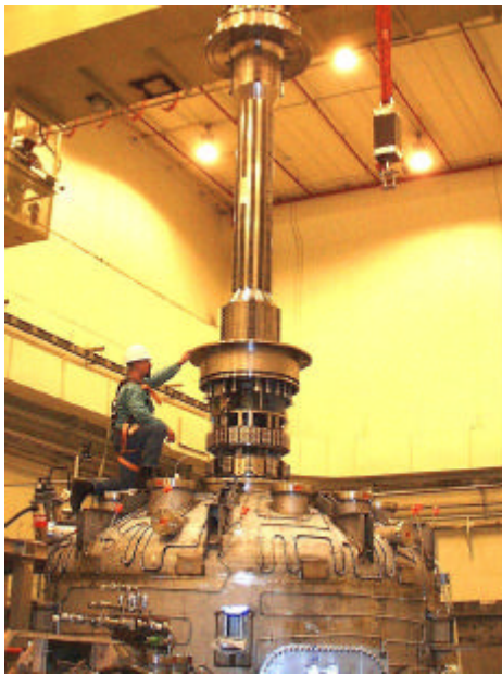
Figure 7- Installation of Centerstack Assembly
