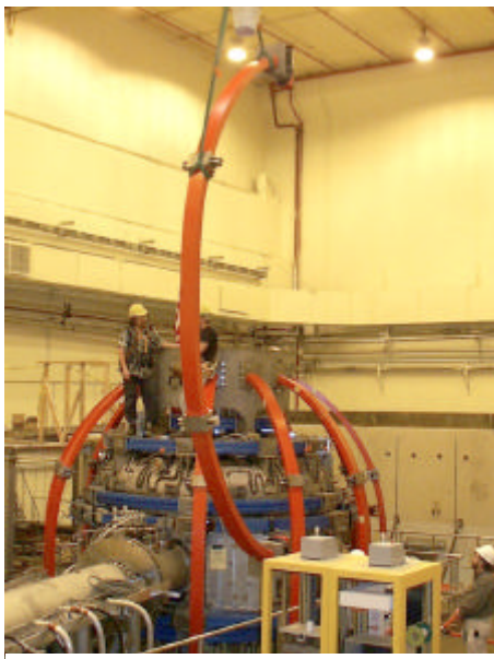
Figure 8- Installation of Outer TF Coil Leg Assembly
