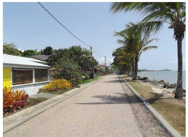
Figure 8: Machans Beach foreshore and rock wall in 2012 (photo Sharon Harwood).
