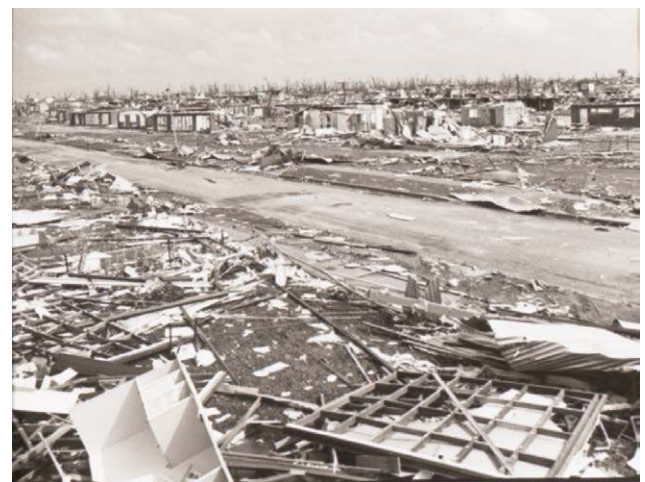
Figure 3: The suburb of Wagaman in Darwin after cyclone Tracy.
