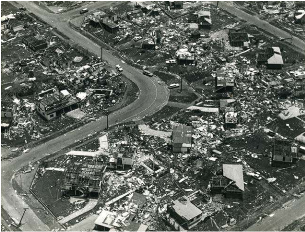
Figure 11: Cyclone Tracy damage in northern suburbs of Darwin.
