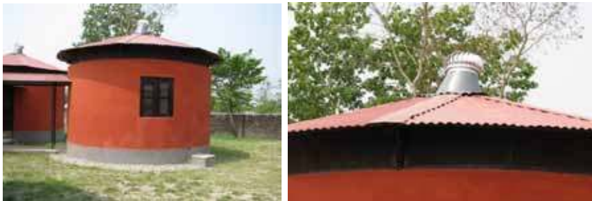
Figure I.2 Individual isolation unit (left), and the gap between the vertical wall and the roof for natural ventilation (right)
