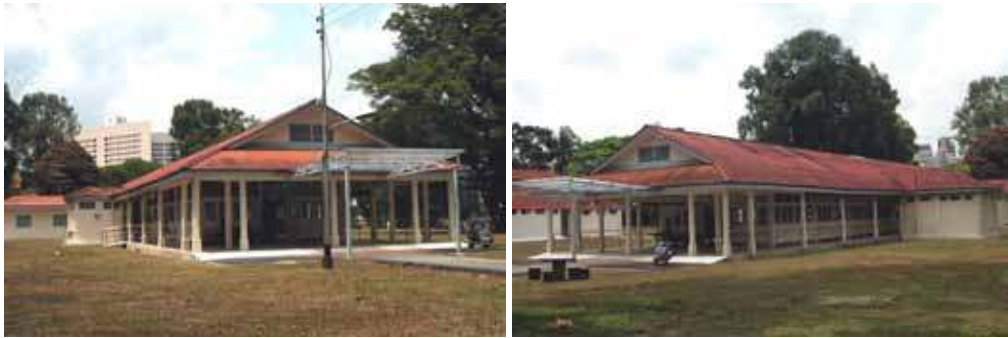
Figure H.1 Two views of the single-storey tuberculosis inpatient ward; the perimeters are free from obstruction, allowing natural ventilation throughout the year
