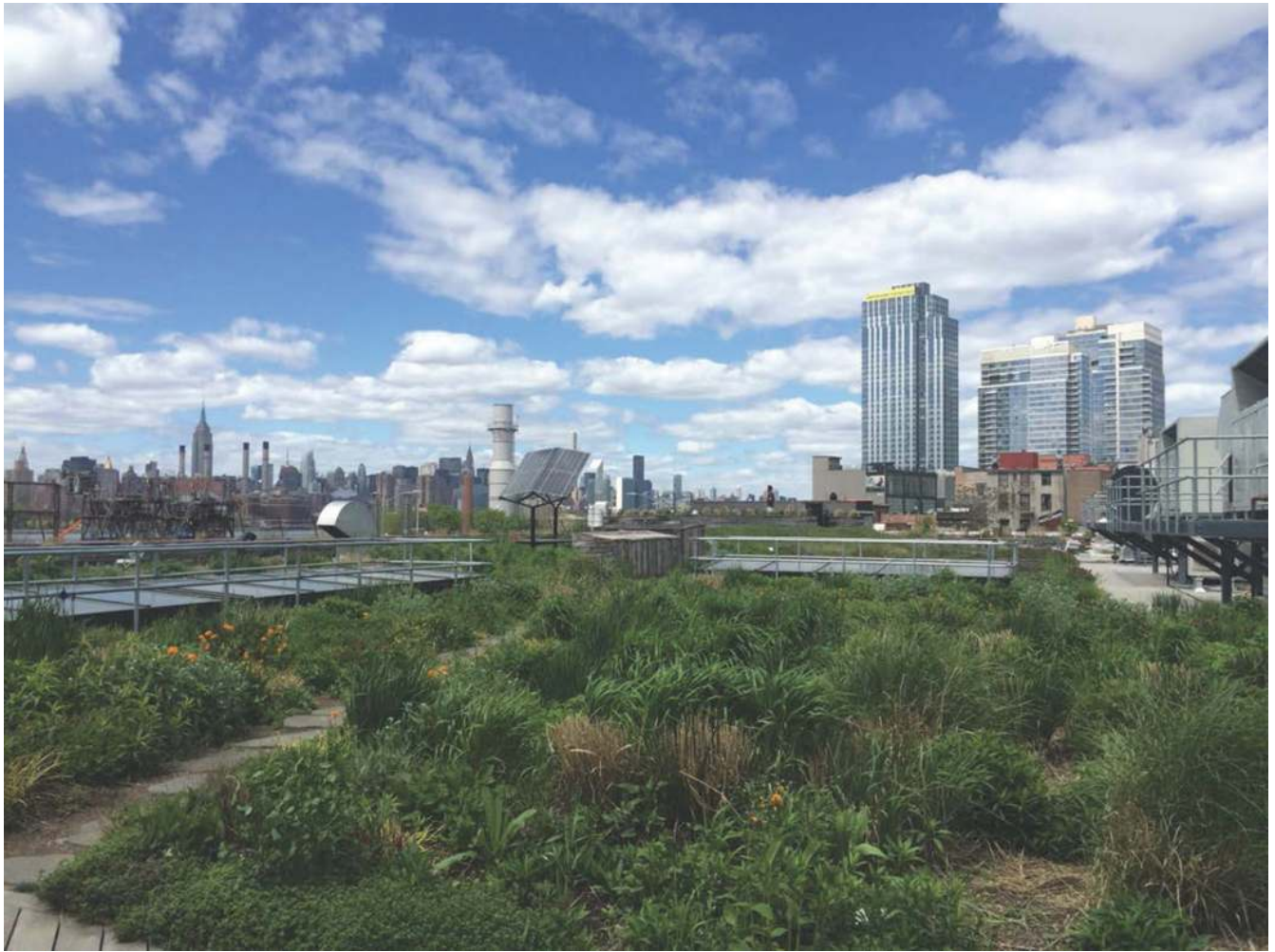
Figure 1. Green roofs are being taken up as nature-based solutions in cities around the world to provide local cooling to mitigate current urban heat islands and projected increases in urban heat driven by climate change (McPhearson et al. 2018). These hybrid green infrastructure systems are also sources for many cobenefits from small- and large-scale food production, to new spaces for recreation and cultural benefits, to opportunities for stormwater capture, habitat for biodiversity and novel spaces for urban environmental education. The green roof pictured here atop the Vice Media Headquarters in Brooklyn, New York, is a biodiverse habitat providing multiple benefits and the site for an undergraduate Green Roof Ecology course at The New School focused on nature-based solutions in urban environments. Photograph: Timon McPhearson.
