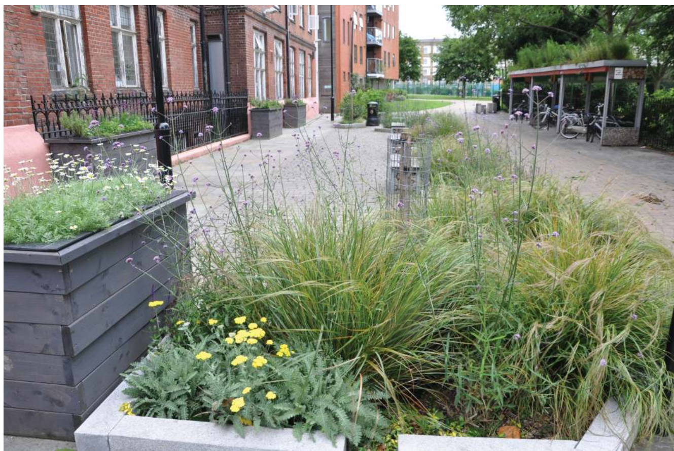
Figure 2. An example of a collection of nature-based solutions to tackle episodic rain but also build cohesion in London. Once a busy road, through the cocreation process it was closed to cars and repaved with permeable paving. Rain is also intercepted from the rooftops of this social housing building in storage boxes and the overflow is then further captured in rain gardens or wild flowers, herbs and insect-friendly plants. More bee-friendly plans can be seen on the roof of the bicycle shelter. The initiative was cocreated to the extent that it is now part of a community interest company (CIC). The CIC manages the nature-based solutions for the local authority and employs several people. There are over 10,000 CICs in the United Kingdom and are an ideal model for comanagement of nature-based solutions. Photograph: Marcus Collier.
