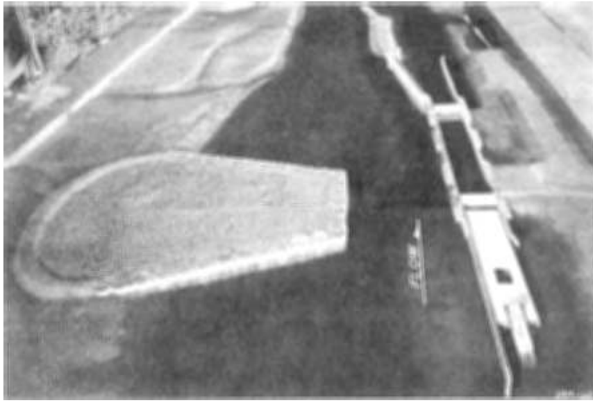
Photo 33. Second-stage cofferdam, Plan D, looking downstream
