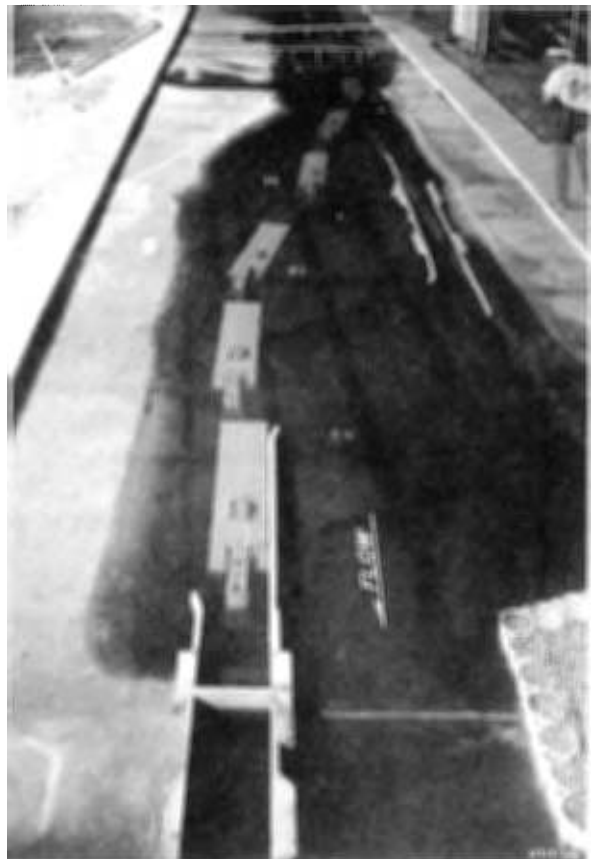
Photo 38. Second-stage cofferdam, Plan D, looking upstream, discharge 60,000 cfs. Path of upbound tow leaving replacement lock
