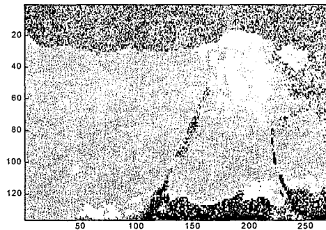
Fig. 6b. Results of the TNDT "tomogram", the gray levels different from the background indicates defects at different depth or cracks
