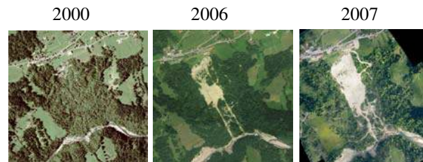
Figure 7 The slope failure in Austria in the years 2000, 2006, and 2007
