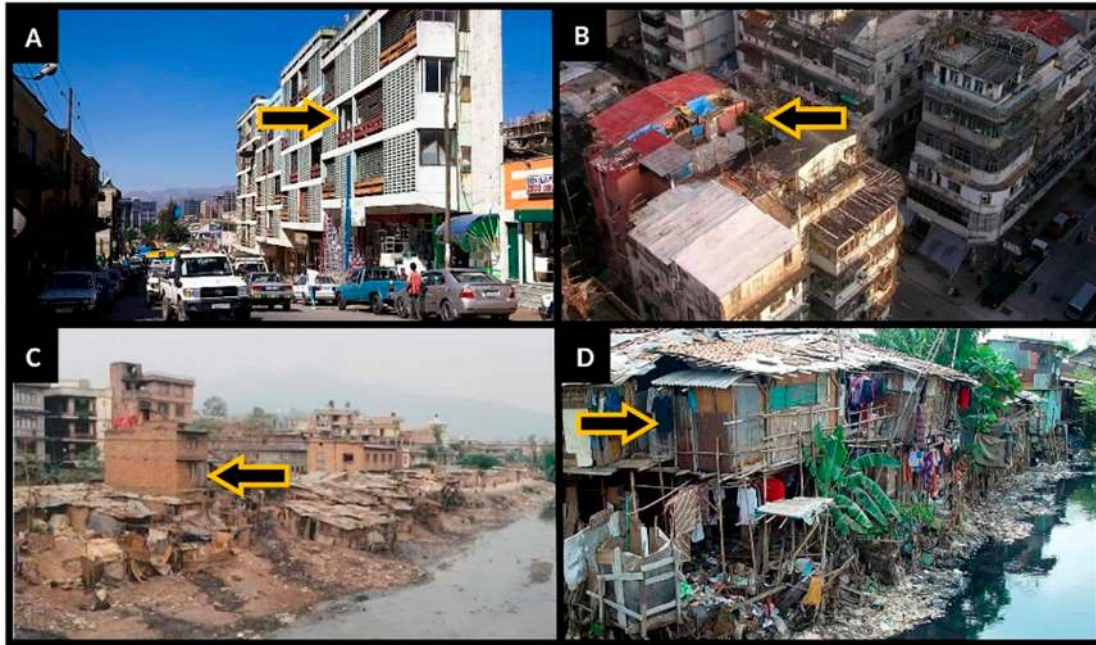
Figure 1. Four ways in which “slum households” and deprived area risk factors intersect. (A) Non-slum household in non-deprived area, (B) Slum household in non-deprived area, (C) Non-slum households in deprived area, and (D) slum households in deprived area.
