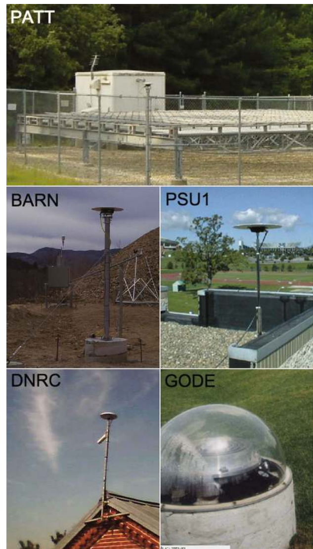
Fig. 12 Examples of station monuments ( http://geodesy.noaa.gov/CORS/ , http://www.profiler.noaa.gov/npn/ ). PATT is located on the corner of a chain link fence. DNRC and PSU1 are installed on metal masts on top of buildings. BARN's antenna is located on a metal mast in a concrete base. GODE is installed on a concrete pillar drilled into the ground
